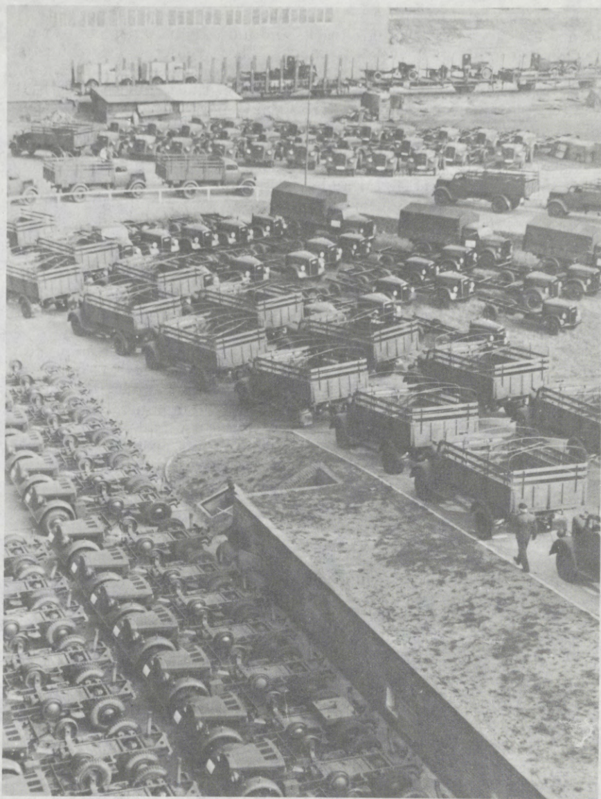
3-TON OPEL "BLITZ" TRUCKS AWAITING SHIPMENT FROM THE GM-BRANDENBURG MILITARY TRUCK FACILITY
