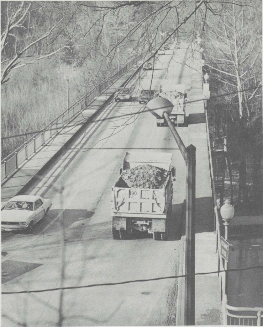
Chain Bridge looking toward Virginia from the District of Columbia. Photo showing heavy load usage. Feb. 10, 1972.
