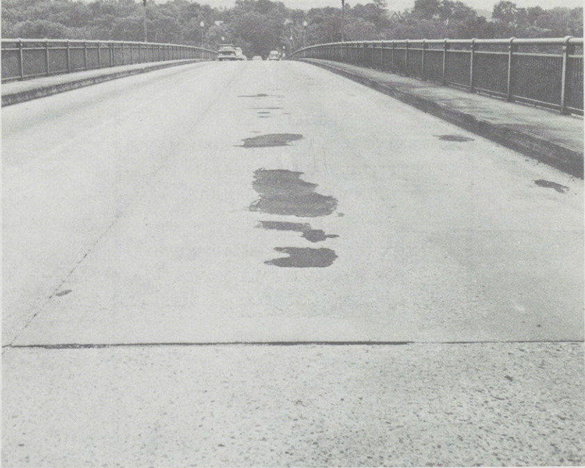
Date: July 29, 1971. Location: Chain Bridge. Subject: Deck condition.
