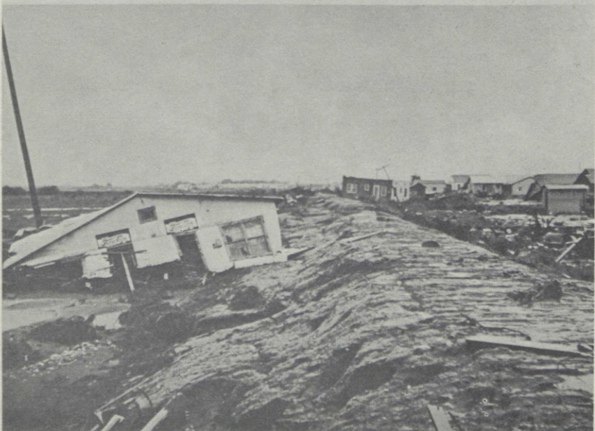
1941 FLOOD Santa Fe main line from Potash Mines washed out
