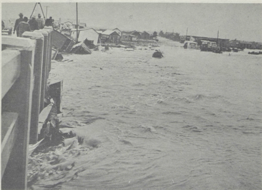
1941 FLOOD High water endangering bridge
