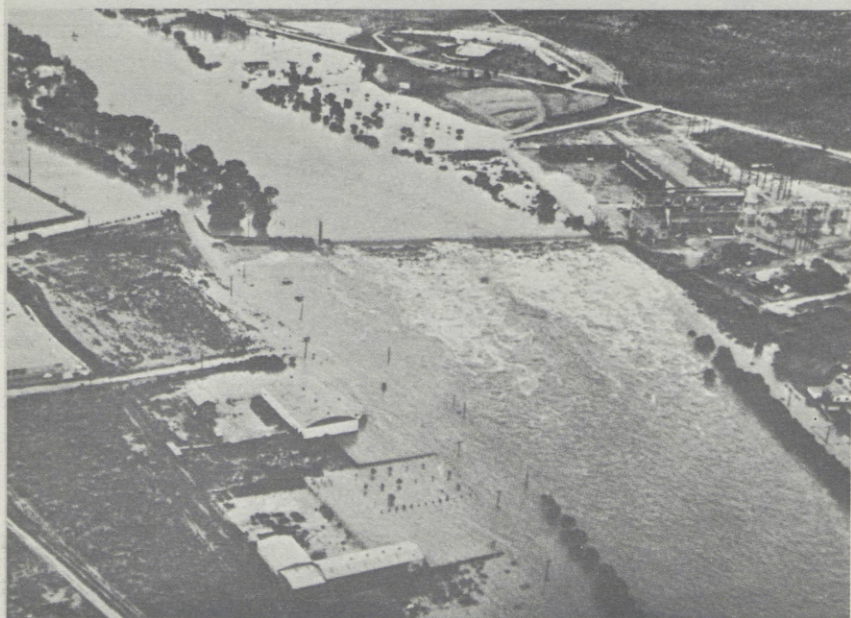
1966 FLOOD Water going over Tansill Dam endangering industrial buildings and flooding recreation area
