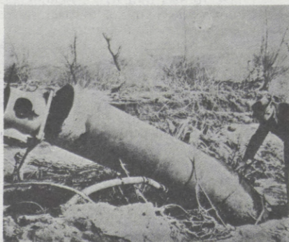
2. Damage to one of principal wells serving Town of Atascadero caused by rampaging Salinas River.
