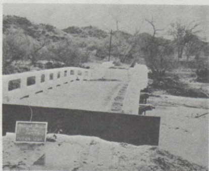
7. Section of bridge destroyed on federally assisted secondary road across Huasna Creek.
