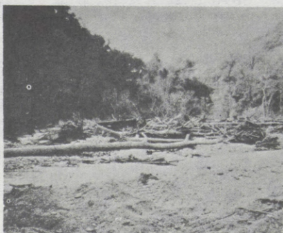
4. Typical debris-filled stream posing major threat to downstream federal, state and county bridges.
