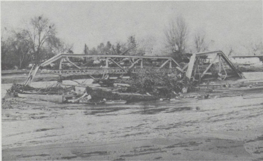
MT. VIEW AVENUE BRIDGE IS CARRIED DOWNSTREAM BY SAN TIMOTEO CREEK
