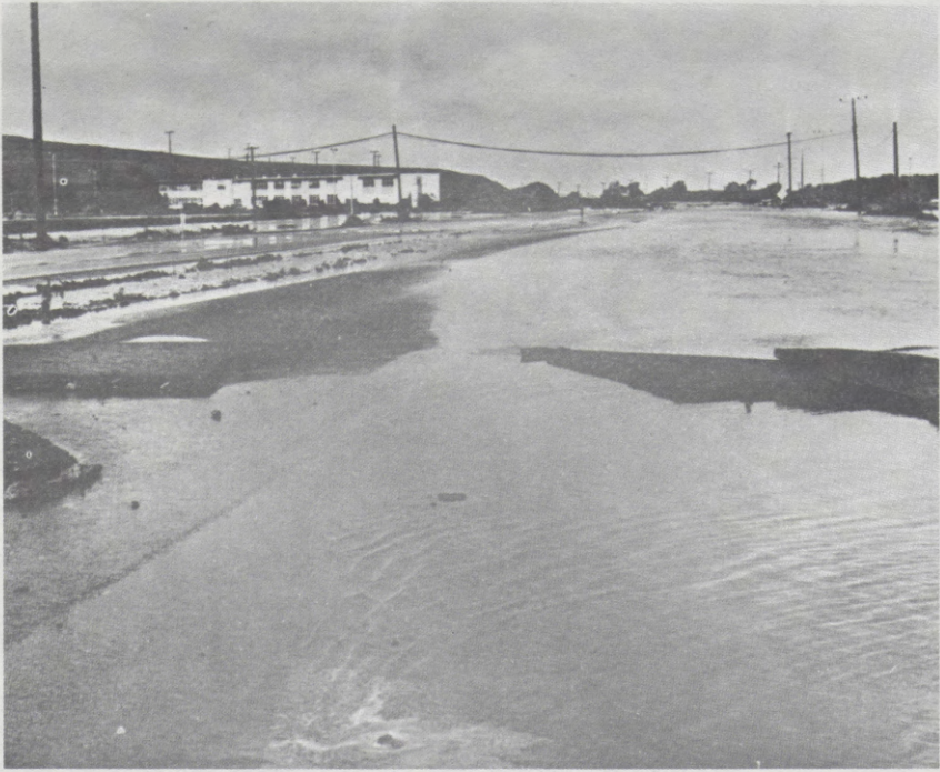
Flooded section of highway near mouth of the Santa Ynez River showing pavement ripped up by flood waters.
