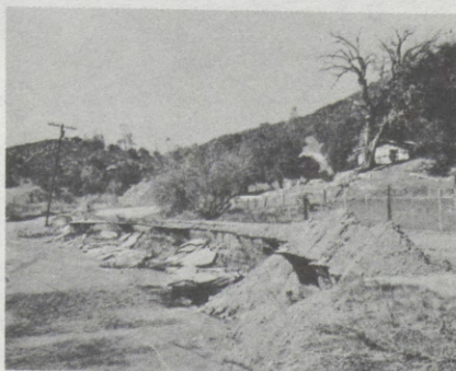
8. Parkhill area road damage, typical of much road damage in San Luis Obispo County.
