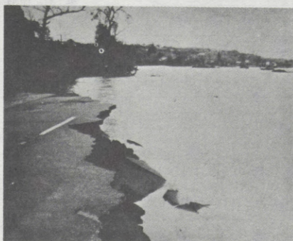
3. Erosion damage to portion of State Highway 41 along Salinas River at Atascadero.
