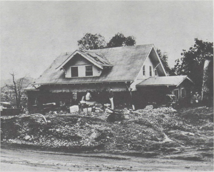
FIGURE 3. Damage from mud and rocks to the Richardson residence, long time residents on Richardson's Hill, Glendora, California. Three to four feet of debris was deposited in and around the building.
