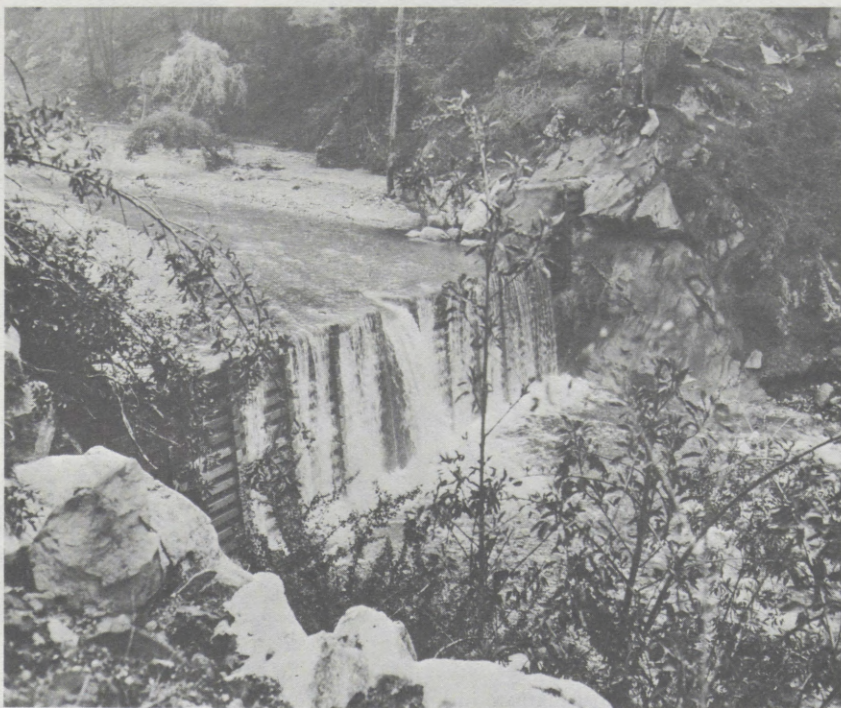
FIGURE 7. Stream stabilization structure limits damage during a storm runoff period. Angeles National Forest, California.
