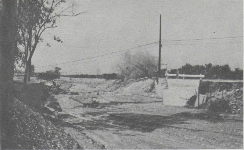
BARTON ROAD, A FEDERAL-AID SECONDARY ROUTE AND MAJOR COUNTY ROAD, LOSES A BRIDGE
