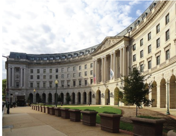
With climate gases emitting from empty offices and dangerous toxins festering in stagnant water, the EPA's headquarters stands as an ironic Washington monument to government teleworking's toll on the environment.
