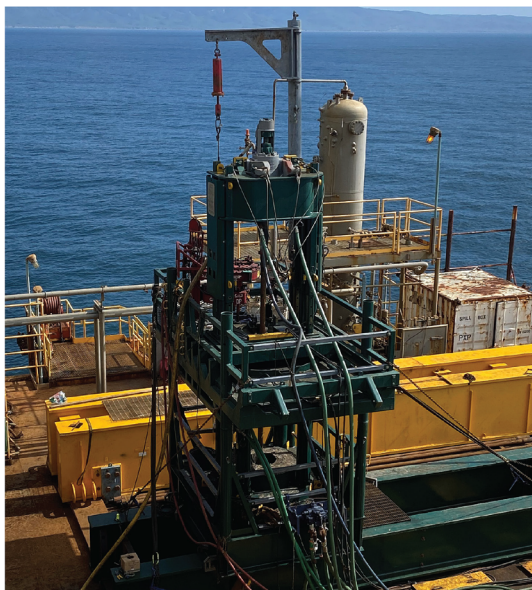
Figure 4: Offshore Well Plugging Operations in the Pacific Region
