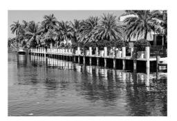
meets the four feet NAVD88 minimum and can structurally support up to 5.7 feet NAVD88 in the future.
