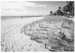
Extensive dune rebuilding efforts were conducted in the aftermath of Hurricane Irma in 2017. The Broward County Shore Protection Project placed 413,000 cubic yaxfo of sand allong the 8.9 miles of shoreline reaching north from Fort Lauderdale, according the U.S. Army Corps of Engineers.
