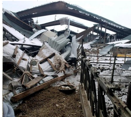
Figure 5 A Dairy Freestall Barn Collapsed due to excessive snow in 2019 in Olmsted County, MN.
