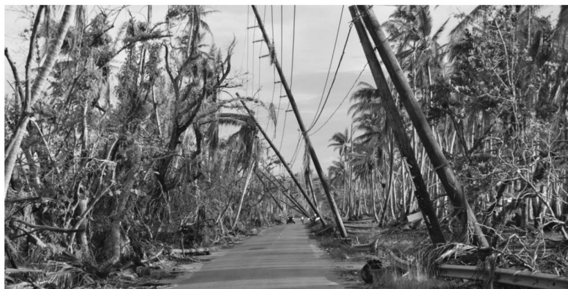
A scene of devastation in Puerto Rico following Hurricane Maria Army Corps of Engineers
