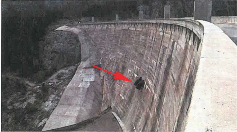
Photo showing two, 6-ft diameter, power penstocks constructed at elevation 4660 to facilitate future hydropower development. Note the top of the concrete wall on the dam crest has an elevation of 4729.
