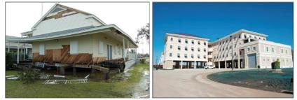
LEFT: Station Sabine Pass, Hurricane Ike, category II damage to station. RIGHT: Station Sabine Pass rebuilt to withstand 100 year flood, category III hurricane wind speeds. Source: U.S. Coast Guard. GAO-22-105513.
