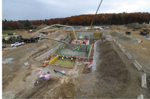
Figure 1: Commonwealth Fusion Systems construction site in Devens, MA (11/09/21)
