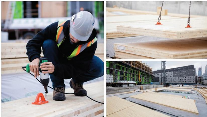
Construction of ARBORA complex with 435 residential units using massive timber in Montreal, Canada. Foto credit: Nordic Structures.
