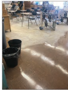
Water damage from HVAC leak in a California school, where officials said repairing flooring is difficult because of asbestos floor tiles. Source: GAO. © GPO 2019-08
