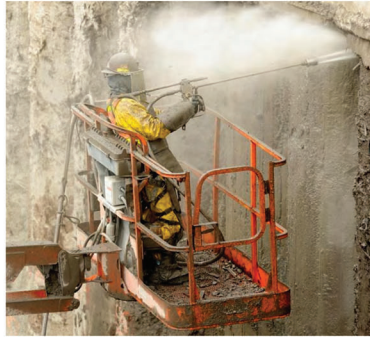
Photo: A Laborer apprentice hydroblasts concrete
