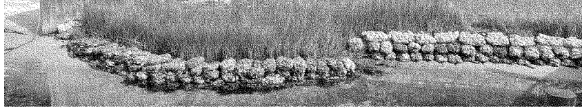
Oyster reef breakwaters and native marsh grasses line a living shoreline in Destin, Florida. Credit: Jennifer McPeak.
