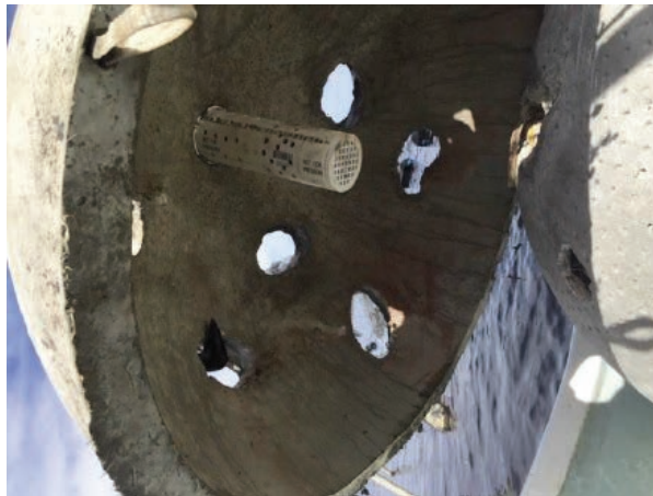
(From the top of the dome, a PVC pipe, holds several mature oysters. The oysters in the pipe spawn and populate the area with oyster that attach to the domes.)
