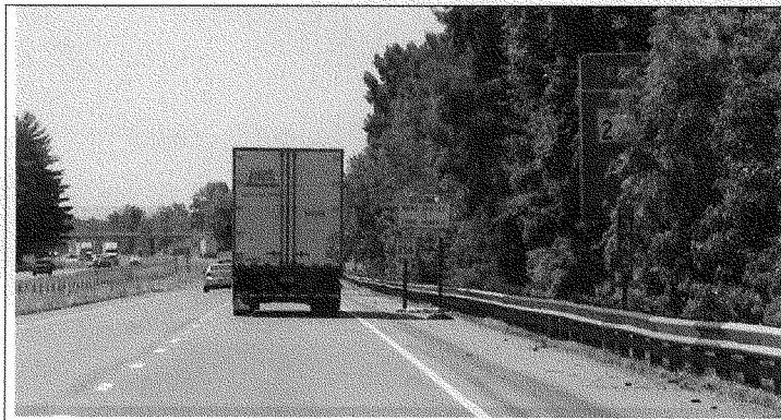
Figure 13: Example of vegetation growth reducing visibility of sign on right side of road
