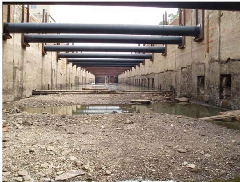
Figure 4—Elizabeth Lock dewatered revealing its deteriorated condition.
