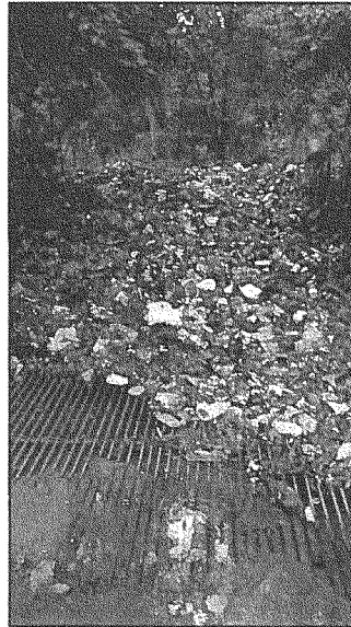
Examples of trash traps installed in tributaries to the Anacostia River in the District. Top: Proprietary device known as a Bandalong Litter Trap™ installed and maintained by Anacostia Riverkeeper. Bottom: custom trash weir designed, installed, and maintained by the Anacostia Watershed Society.
