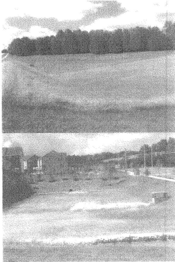
The above two pictures show dry temporary detention areas that could be built in the BGE right of way. The top one is on Union town road, a three acre mowed field, the road is the dam, the riser is in the middle left, 12 acre feet of storage, efficient and inexpensive compared to the ones I've seen in the Hydrology study. The bottom is in front of Lyons Mill elementary in Owings Mills, both only become wet in heavy rain, hours later they are dry.
