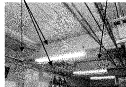
Expanding cracks in the ceiling support beams
