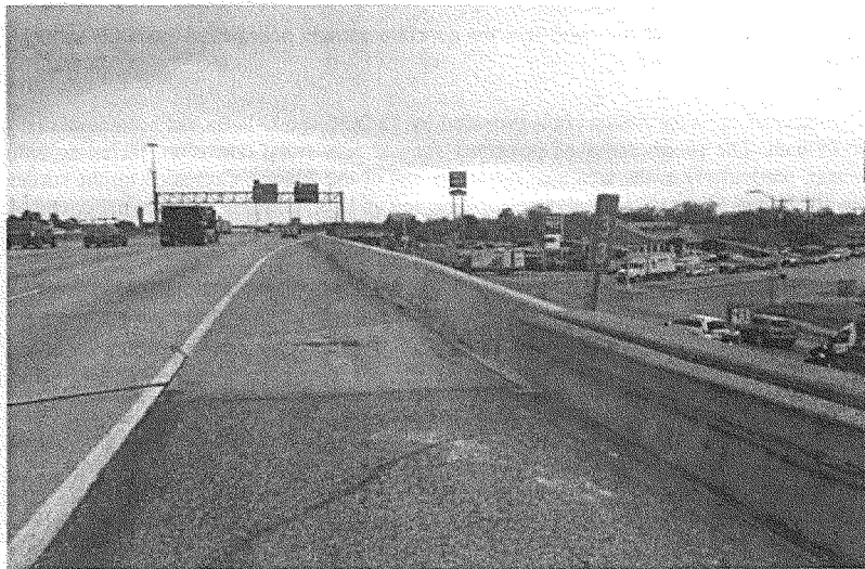
Figure 8. Looking to the southeast along the new single-sloped concrete traffic rail installed by the TxDOT Houston District after the crash. (Source: TxDOT Houston District)
