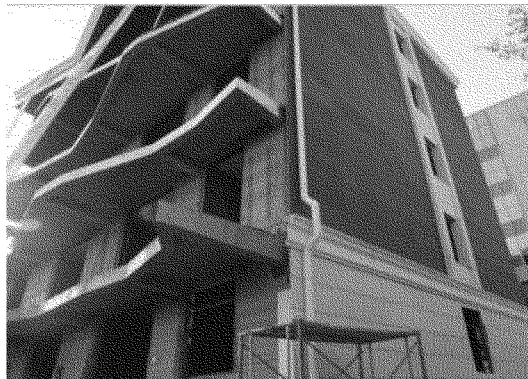
Figure 15: 6-story 3D printed apartment building (Sevenson, 2015)
