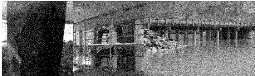
Figure 12. Rehabilitation of corroded steel H-pile bridge using composites, East Lynn Lake Bridge, East Lynn, WV. The repair cost 35% of the cost of a conventional repair. (WVU, 2014)
