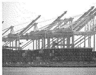
Port of Oakland cranes Photo: Steve Belmont, http://www.danah.com/
