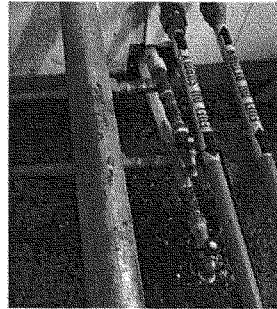
Refitted transition to HEPex
