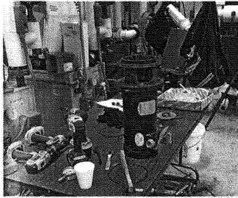
Loop 1 - #2 circulation pump - seal kit installation
