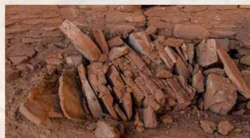
Wall knocked down by careless visitor or possibly a cow.
