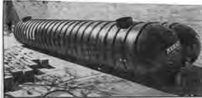
ABOVE: The landscaping makeover at the court building includes large underground cisterns to capture rain water from the roof and grounds to irrigate new plants and trees.
