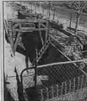
ABOVE: The landscaping makeover at the court building includes large underground cisterns to capture rain water from the roof and grounds to irrigate new plants and trees.
