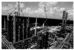
Southern's Kemper Project in Progress: "The Kemper plant will use two commercial-scale TRIG™ units to gasify lignite (low-rank coal that is mined next to the facility) to produce syngas. After the syngas leaves the gasifiers, it will be cleaned and used as fuel for two combined-cycle power generating units with a net output of 582-megawatts of electricity." Global CCS Institute Status of CCS.
