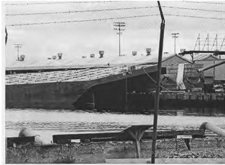
Senator MENENDEZ. In Jersey City, a float used to move railway cars broke in half and created significant damage. 150 feet of railroad track was washed away. Cargo-handling cranes and other pieces of equipment were severely damaged.
