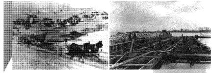
ABOVE, FROM LEFF: Early levee construction, around 1910. Workers construct a willow mat that will be loaded with rock for channel protection or wing dike formation.
