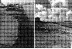
EAR LEFT: Post-flood cracking of the concrete at the Baton Rouge waterfront. LEFT. The same shot after stabi-lization with rock.
