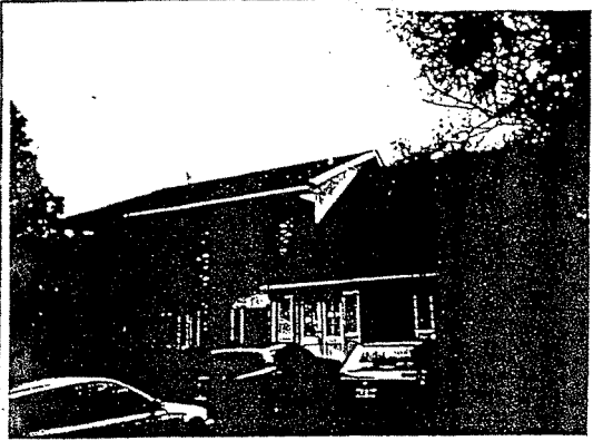
FRONT OF SUBJECT PROPERTY
