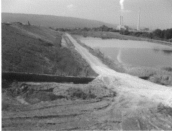
Photo A-1: As Found Site Conditions of the West Slope of Gypsum Stack; Process Water Redirected Through Temporary Spillway Discharge Pipe (foreground)
