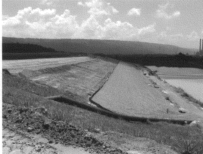
Photo A-3: Completion of Rock Toe Buttress and Preparation of Vegetative Cover Along the West Slope of Gypsum Stack
