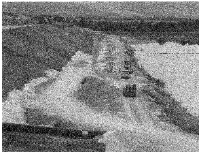
Photo A-2: Construction of Rock Toe Buttress and Spillway Renovations Along West Slope of Gypsum Stack
