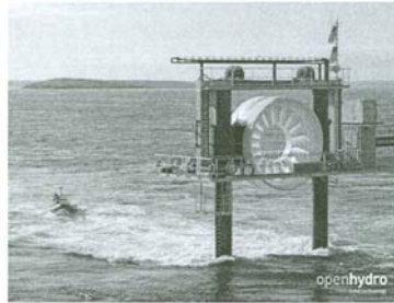
Figure 2: OpenHydro Research and Development Installation
