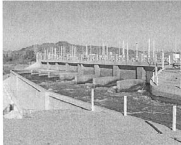
Gila Gravity Canal Headworks; 2,200 cfs max flow; 14 feet head; 2.4 to 5.9 MW potential
