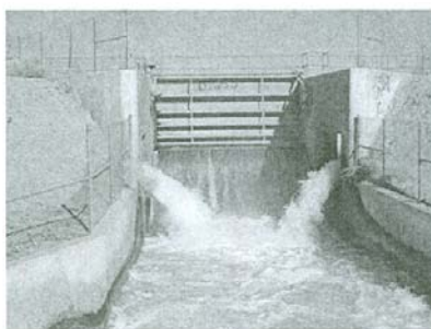
Maricopa-Stanfield Irrigation District Drop Structure; 100 cfs; 10 feet head; 200 kW potential
