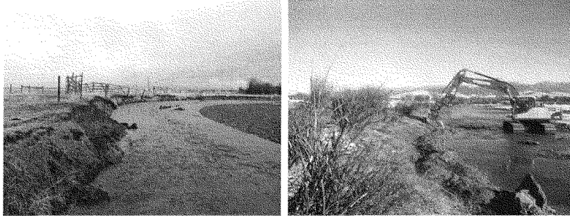
Pre-Project streambank in need of stabilization compared to post-project streambank after stabilization with toe slope armoring, willow planting, and sodmats.
