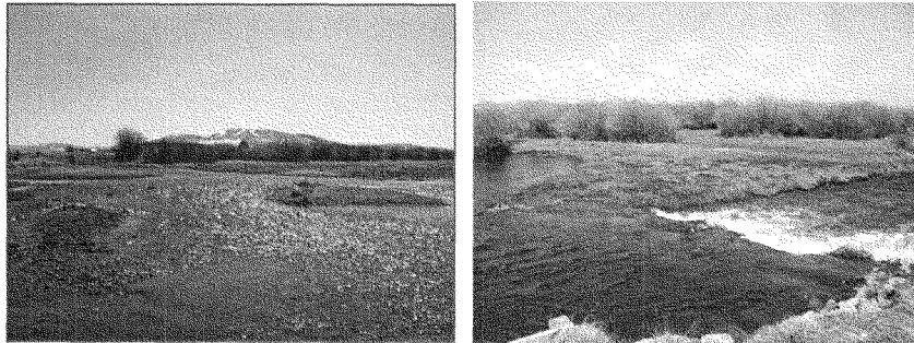
Jackson Reach Project Site: Pre- and post-project. Water gap partially restored by development of point bar
