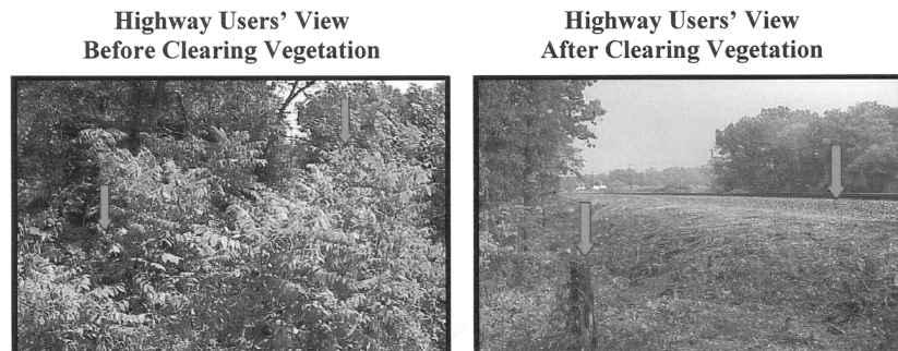
Figure 1. Photographs of Highway Users' Line of Sight at a Grade Crossing Before and After Vegetation Was Cleared
