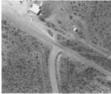
Skewed intersection at IRR Route 15 and State Route 86. Source of the aerial photo is Google Earth.
