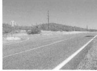
State Route 86 looking east and north. Photo taken by ITCA. Provided courtesy of TON.
