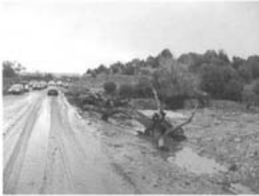
Fort Apache Reservation. Example of debris, mud and water on a roadway that resulted from a normal 2004 monsoon. Provided courtesy of BIA Fort Apache Agency.
