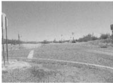
State Route 86 looking eastbound. Photo taken by ITCA. Provided courtesy of TON.
