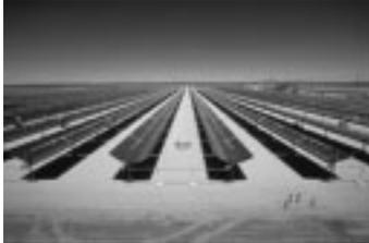
Concentrating solar power (CSP) plants are utility-scale generators that produce electricity by using mirrors or lenses to efficiently concentrate the sun's energy. Two principal CSP technologies are parabolic troughs and dish-Stirling engine systems.
