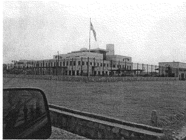
Bureau of Overseas Buildings Operations (OBO) "Standardized Embassy Design" (SED) U.S. Embassy, Bamako, Mali
