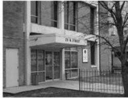
CSOSA Field Office at 25 K St NE.
