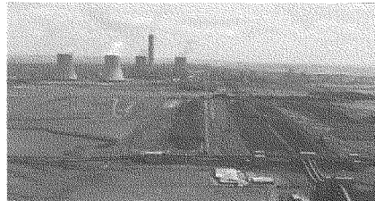
Coal liquefaction is proven technology that has been enhanced by modern research. South Africa's SASOL Co. developed a commercial coal liquids industry that produces about 135,000 barrels daily at its Secunda plant.
