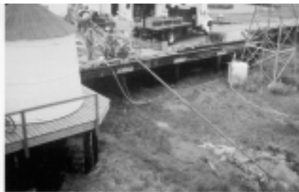
Above, LEO's cable from the field station is directionally drilled underneath a moored and instrumented submersible and toward the continental shelf. Below (top to bottom), the WHOI designed remotely operated vehicle ROPOS observes Environmental Monitoring Unit's, an underwater docking station where ROPOS can upload power or download data, and of LEO's seafloor nodes in deployed
