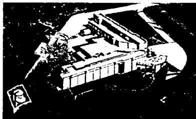
DARHT at Los Alamos. The Dual-Axis Radiographic Hydrodynamic Test Facility, currently under construction, will provide experimental data on the implosion phase of nuclear warhead operation.
