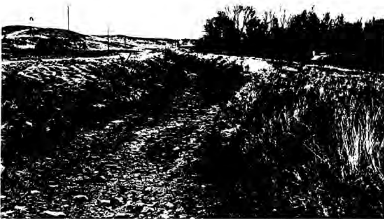
Johnson Lateral - Beginning of 12 mile Lateral - High loss lateral. Runs through gravelly soils. March, 1994 photo.
