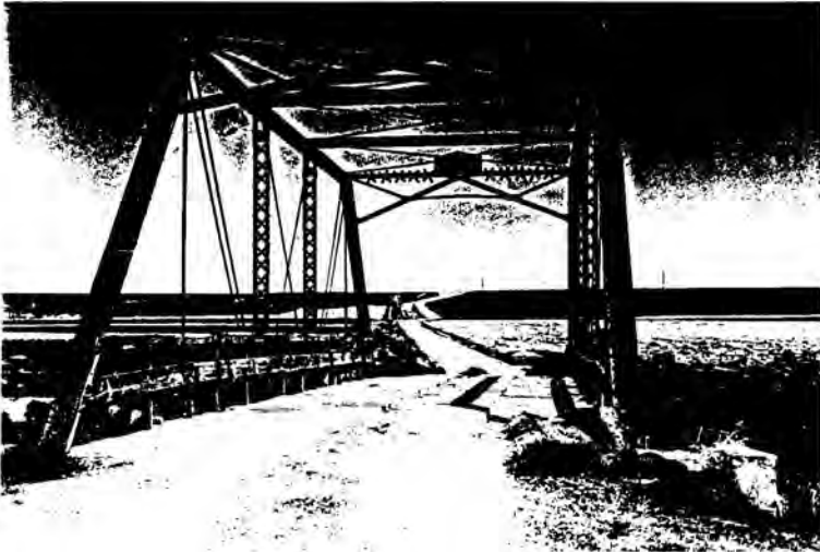
Bridge No. 3 - On Inlet Canal, one of the Court Case Bridges. Located S4 Sec 29, T9N - R3E. 5/18/93.
