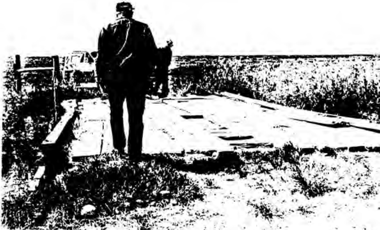
Bridge No. 88 - Bridge located on the N. Bdry. NE4 Sec. 9, T9N, R5E. 5/18/93.
