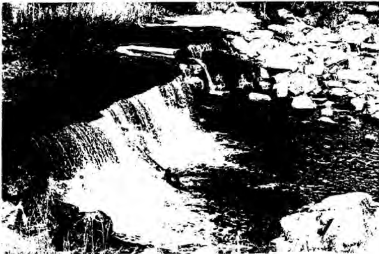
Whitewood Creek Siphon. Side view. September, 1993.
