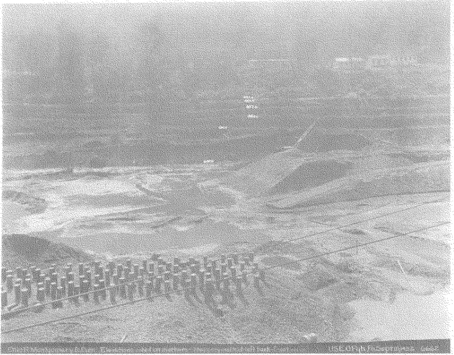
Photograph 1. Overview of Montgomery Dam Construction. View to South. Note construction buildings in background. (Photograph Courtesy of USACE, Pittsburgh District.)
