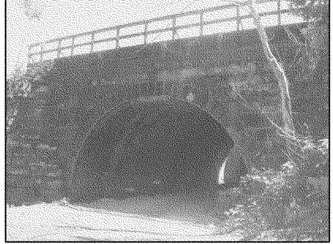
Photograph 12. Railroad Underpass. View to North.
