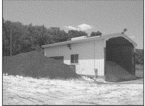
Photograph 15. Road Maintenance Structure. View to South.
