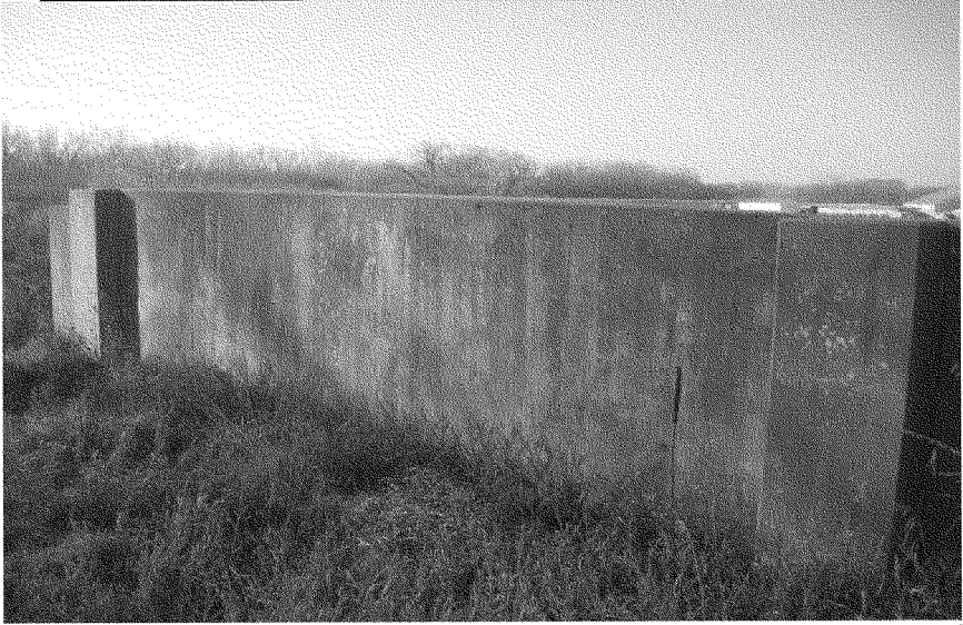
Figure 1: Riverside face of former stop log gap Sta. 83+24 prior to placement of fill.
