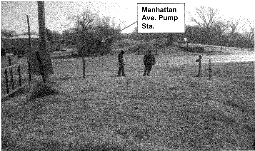
Figure 4: Sand Bag Gap at Sta. 20+00 Standing on right abutment (if viewed from landside). Gap extends across Manhattan Ave. to left abutment across street. Manhattan Ave. pump station in background.
