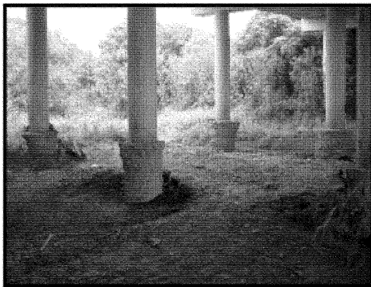
Culebra Creek - Culebra St Bridge Piers Scouring
