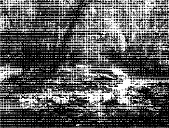
Photograph 1: showing upstream location with existing weir cut out and rubble to be removed
