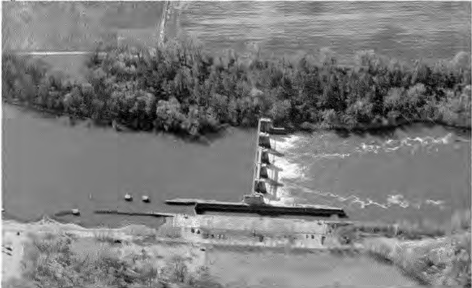
Figure 8.1.2-1: New Savannah Bluff Lock & Dam
