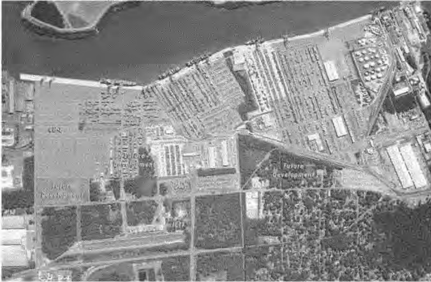
FIGURE 2 GARDEN CITY TERMINAL – AERIAL PHOTO
