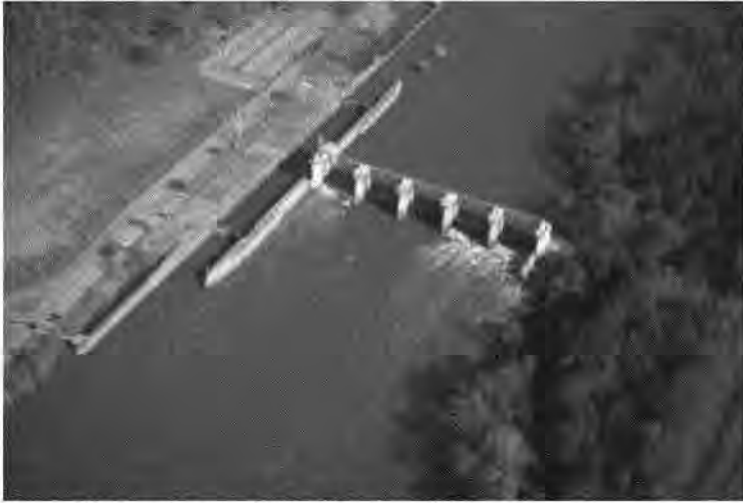
Figure 22. New Savannah Bluff Lock and Dam
