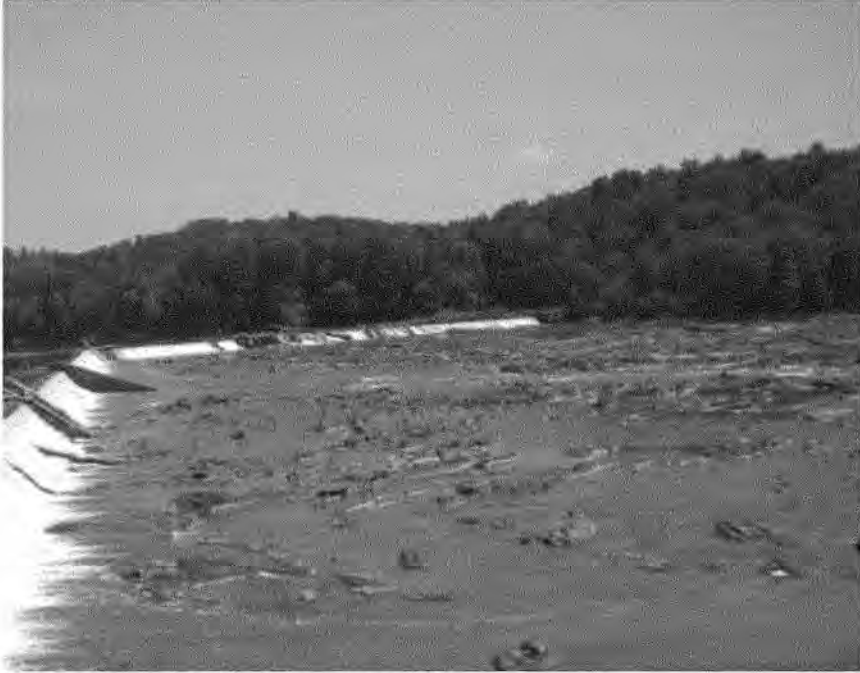
Figure 24. Augusta Diversion Dam and Shoals
